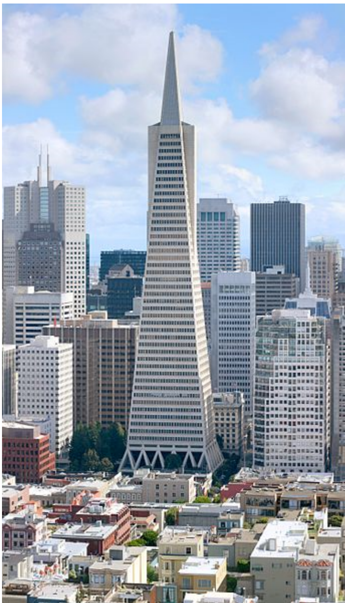
Figure 5. San Francisco Transamerica Pyramid Building. Source: authors.
